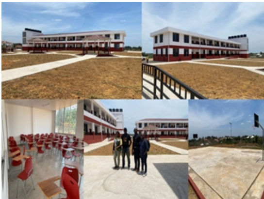
Completed Francis Lewis Morris Modern Secondary School, Kakata City, Margibi County
