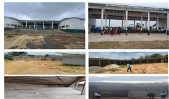
Completed CARI Agricultural Mechanization Service Center, Suakoko, Bong County (Upper Right and Left) and ongoing Construction of Kolahum & Foya, Lofa; Kakata, Margibi and Gbedin Nimba Counties Agricultural Mechanization Hubs (Bottom)
