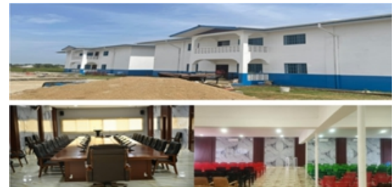
Ongoing Renovation and Rehabilitation Liberia National Police Training Academy Hospital (Above) and Completed Conference Room Facilities (Below)
