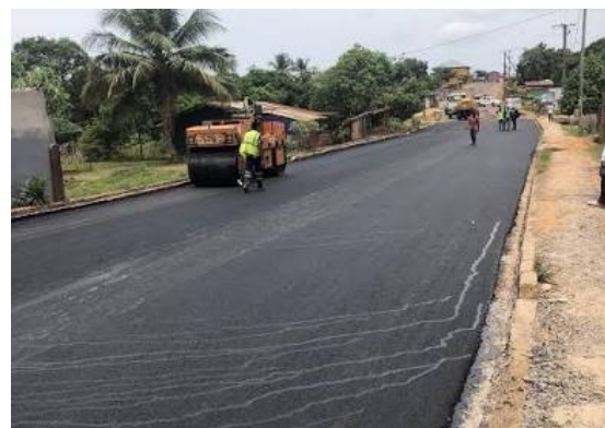
Soul Clinic, Paynesville Road construction
