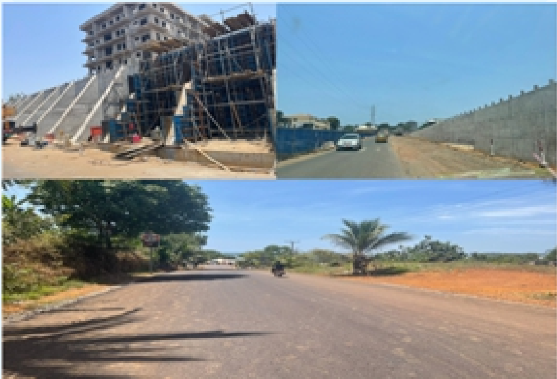
Ongoing Ministerial Complex & SKD Boulevard Bye-Pass Chinese Aid Project 2- Overhead Pass Bridges (above) & Robertsport - Medina Road (below)
