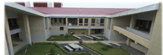
Ongoing Reconstruction of C.H. Rennie Hospital, Kakata City, Margibi County (above) & Newly Constructed Redemption Hospital, Montserrado County (below)
