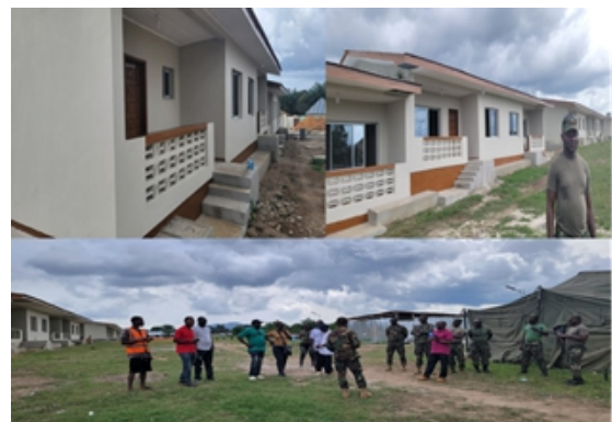
Completed & Commissioned Rehabilitated Camp Grant Military Barrack, Sanniquellie City, Nimba County
