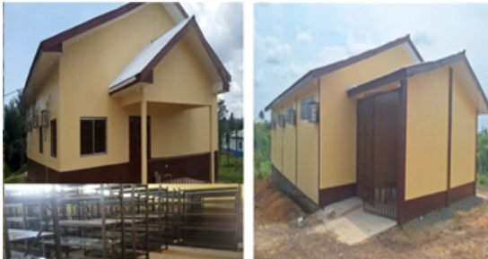
Completed Grand Kru County Drugs Depot/Warehouse, Barclayville City, Grand Kru County (Left) and Bong County Drugs Depot/Warehouse, Gbarnga City, Bong County (Right)
